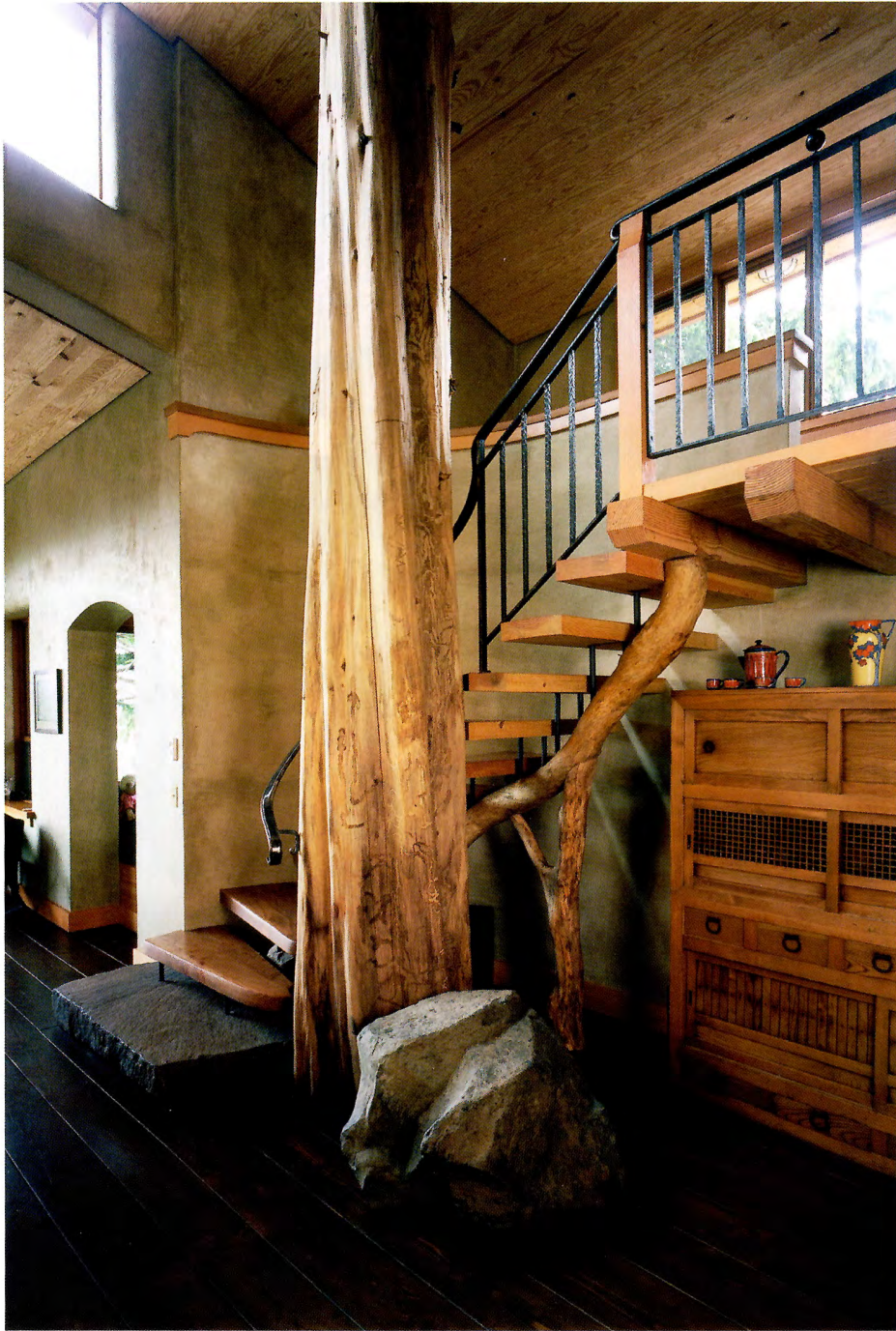
Above: Windfall-harvested Douglas fir is used for the stair planks and much of the flooring. A large tree trunk forms an interior feature and was actually found on site. The interior walls are covered with gypsum plaster. These were soaked and covered with Aglaia – a natural, aromatic pigment.
