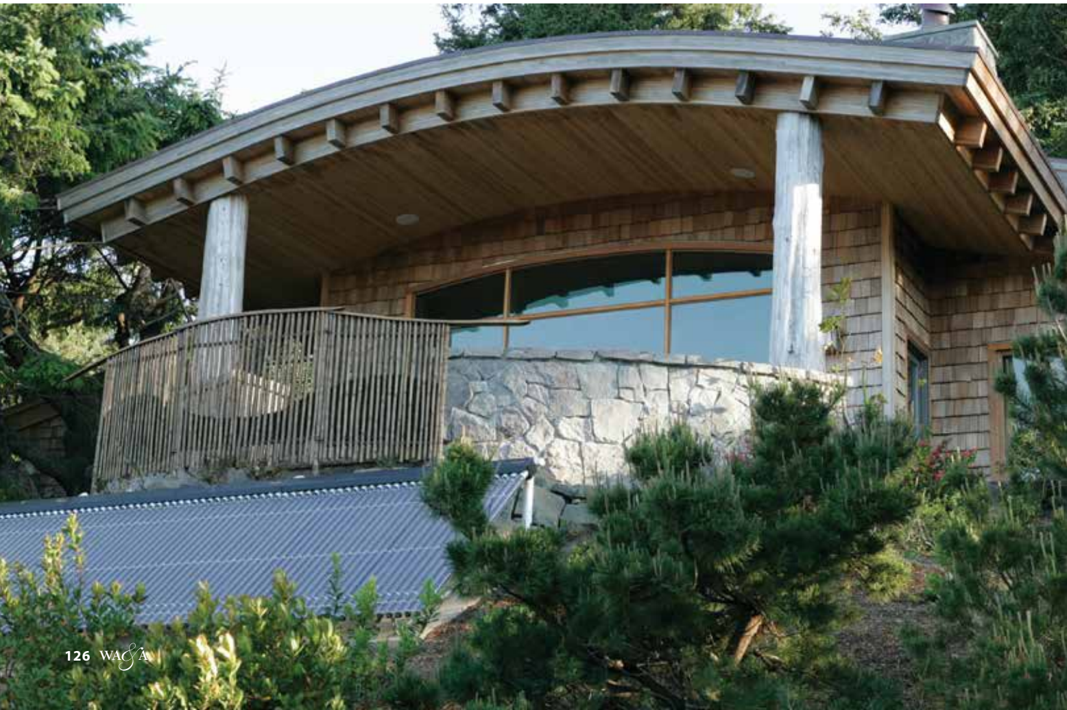
From top: A wooden sculpture anchors the hallway. | Two incense cedars serve as natural columns to support the south-facing covered porch. The bamboo privacy screen was designed by Shannon Belthor. An evacuated tube solar-thermal system provides heating and hot water to the house. Photos: Greg Kozawa
