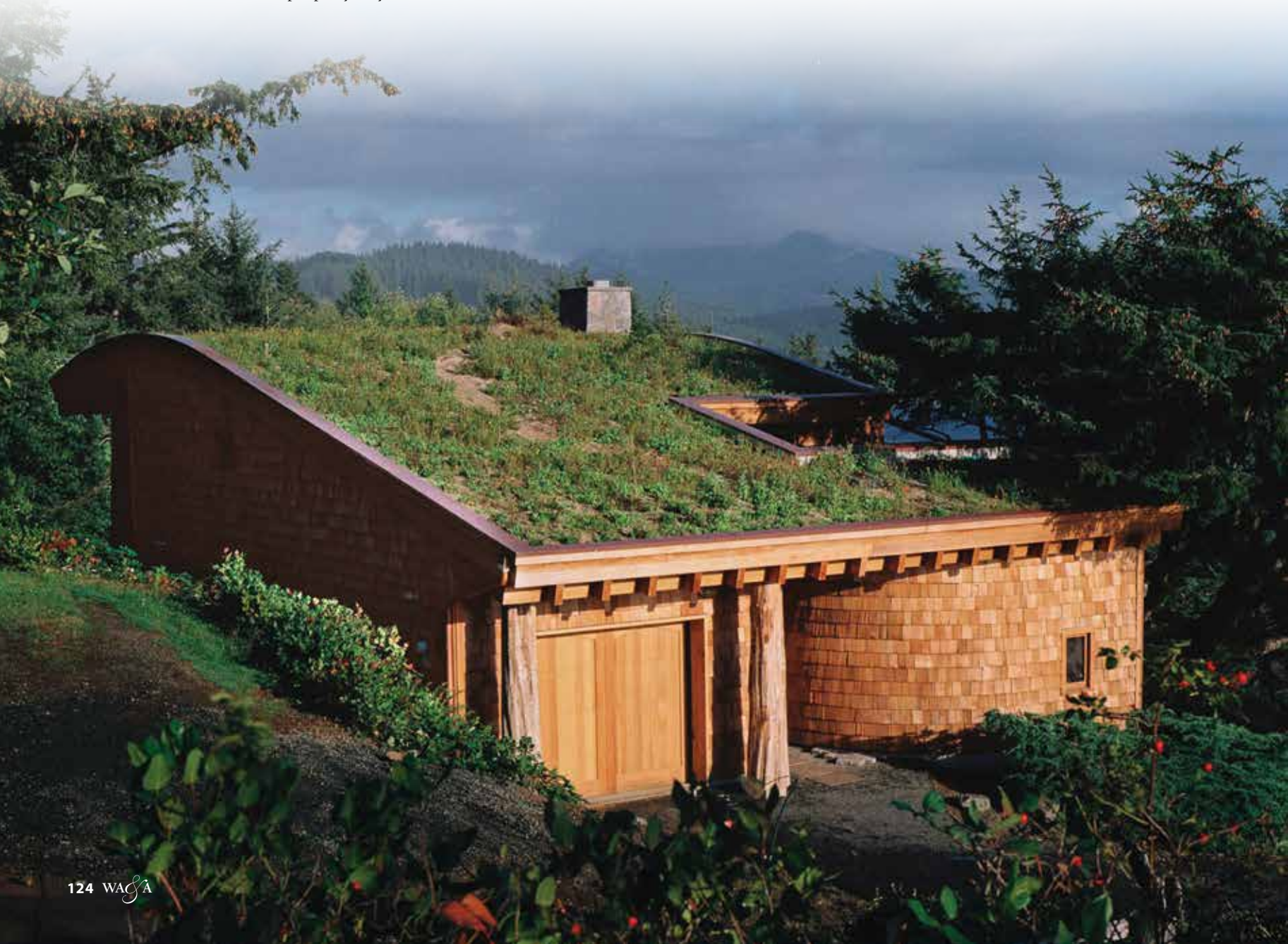
This page, from top: The dining room at the Cannon Beach House features a live-edge table of wind-topped Douglas fir. The same wood forms the heavy timber frames in the Camas Basalt thermal storage wall. | The green roof softens the view of Cannon Beach for the houses above it and reduces the rate of rainwater flowing into the neighborhood stormwater system. The home was designed around an ancient Sitka spruce, and the Western red cedar shakes were sourced from an Audubon forest in Washington. Photos: Nathan Good Opposite page: An incense cedar column anchors the staircase, which leads to a loft. The stair treads are wind-fallen Douglas fir, and the boulder was originally meant for a fireplace but was too heavy to move after it was rejected. Photo: Daniel Root
